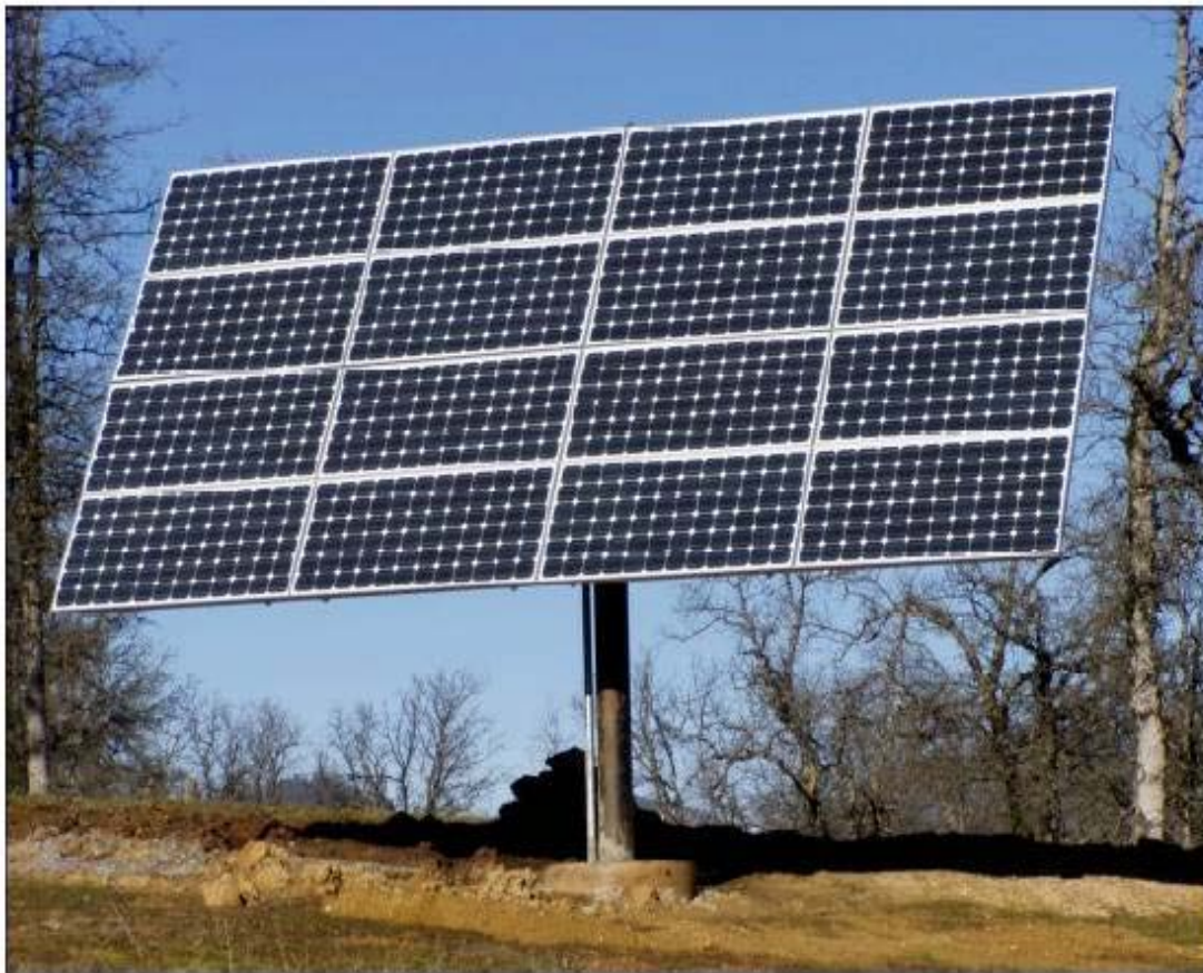
Sixteen, BP 150 watt modules mounted on a Wattsun AZ-225 Tracker Drive.
